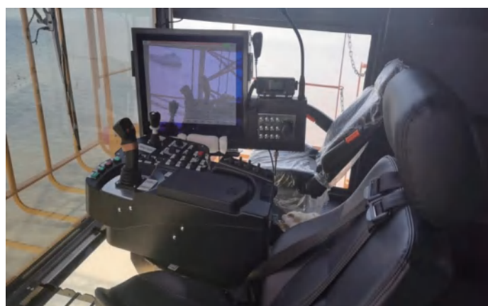
(Crane Operation Chair&HMI)
